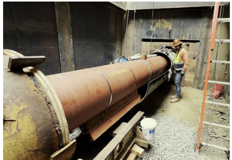
18-inch NO-DIG Pipe installed within a 36-inch steel casing in Ontario, CA
