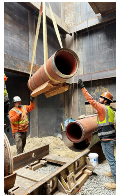
2M section length of 18-inch Vitrified Clay Jacking pipe with redwood skids being lowered in a jacking shaft
